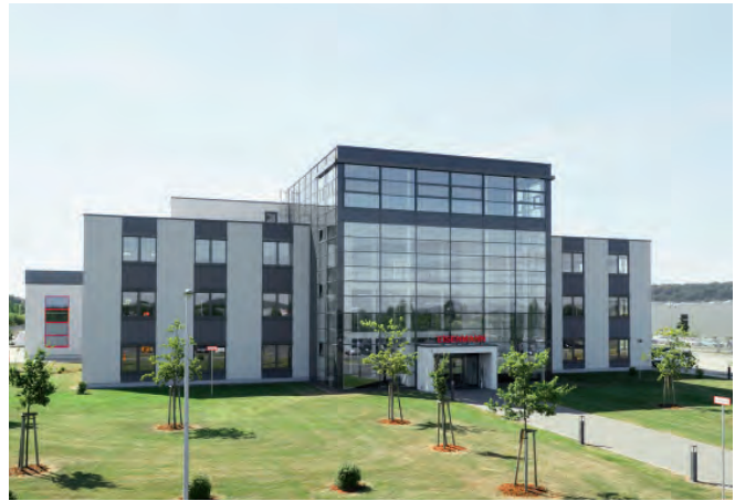
Ruhstrat/Eisenmann Thermal Solutions in Bovenden
